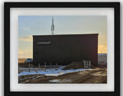
Landsnet hf. Vegamót - Tengivirki
